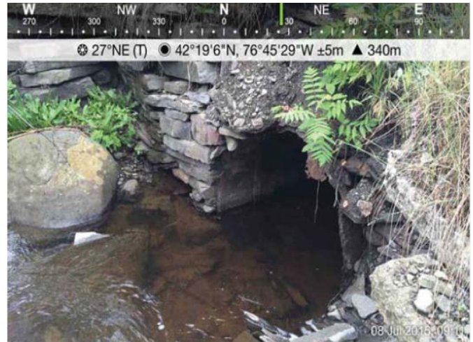
Culvert under Pertl Road, August 2015 photo credit: Schuyler County Emergency Management
